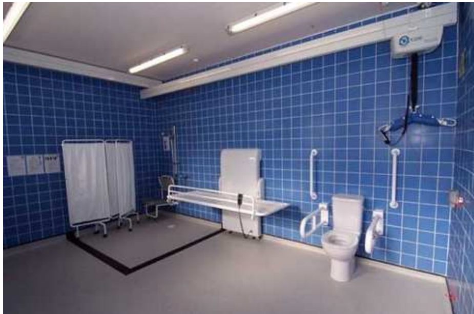
Fig 2.14: Fully accessible toilets with high footfall
