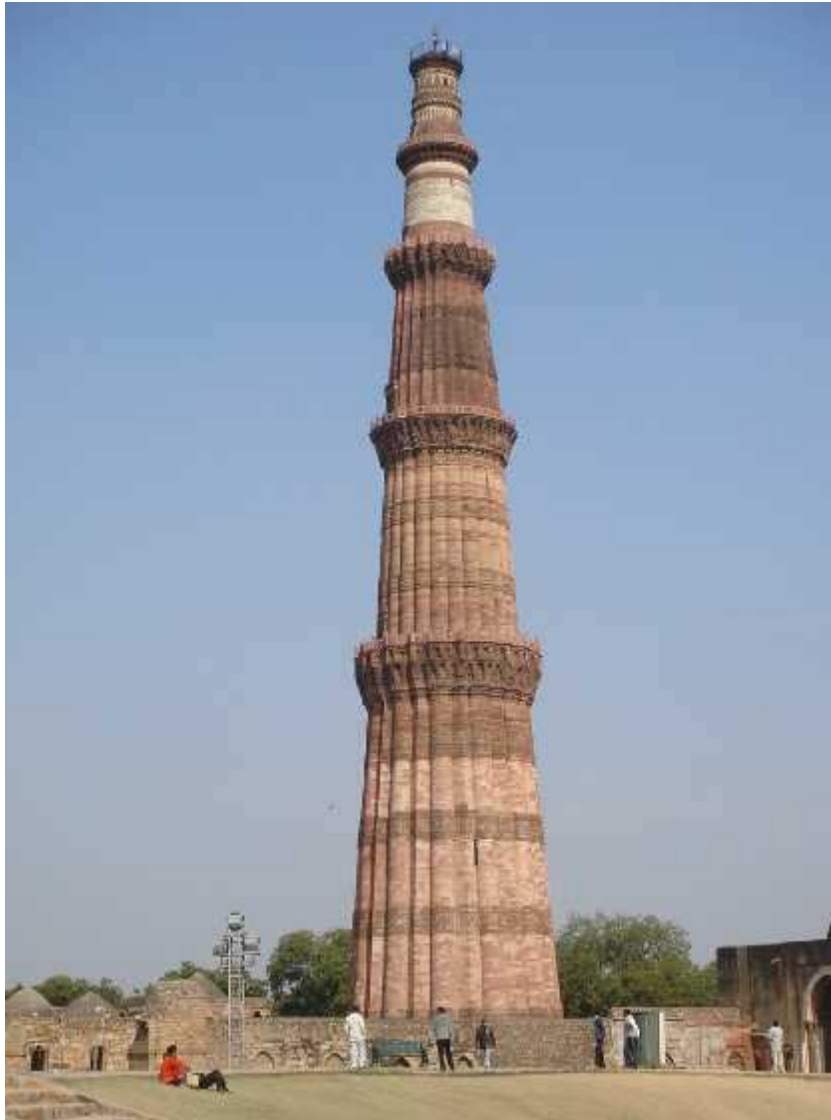
Fig 1.07: Qutb Minar (Delhi, India) Qutub Minar is a 73-metre (239.5 feet) tall tapering tower of five storeys, with a 14.3 metres (47 feet) base diameter, reducing to 2.7 metres (9 feet) at the peak. It contains a spiral staircase of 379 steps.
