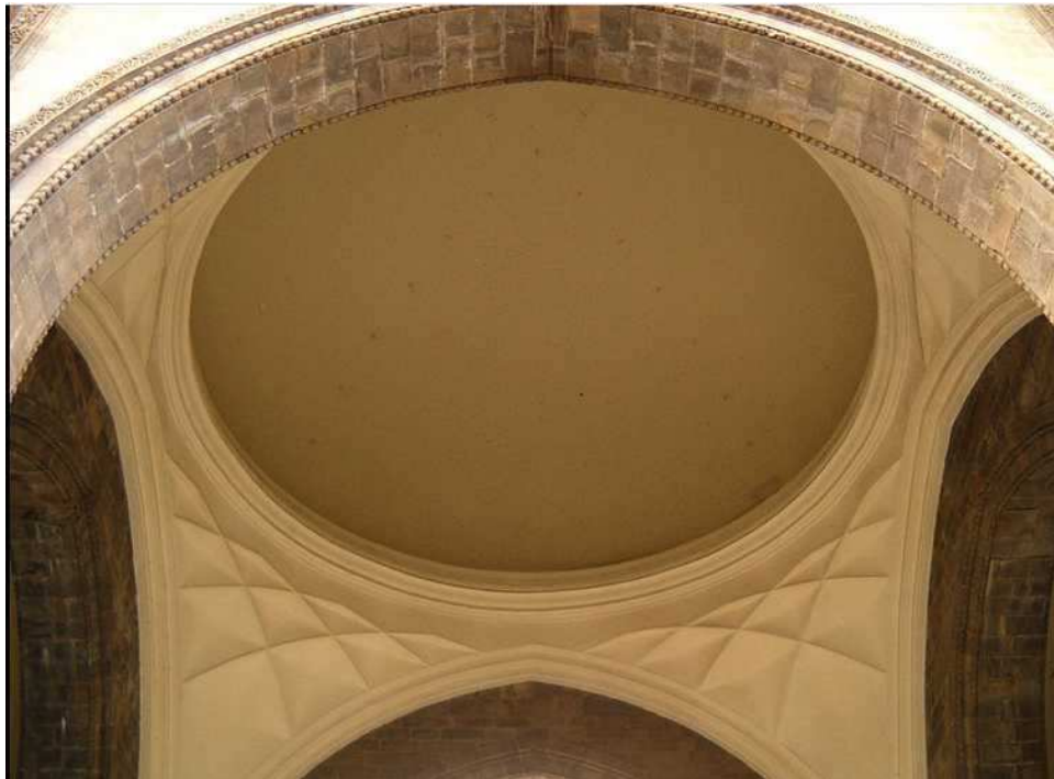
Fig 3.30: Internal View of the Dome
