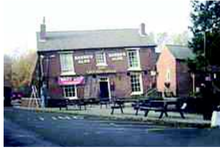
Fig 3.14: 'The Crooked House', Himley, is known for the extreme lean of the building, caused by subsidence produced by mining
