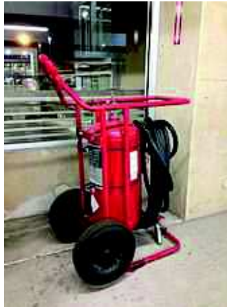
Fig 2.13: Wheeled fire extinguisher and a sign inside a parking lot
