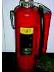
Fig 2.23: Ansul Met-L-X 30lb. cartridge-operated sodium chloride dry powder
