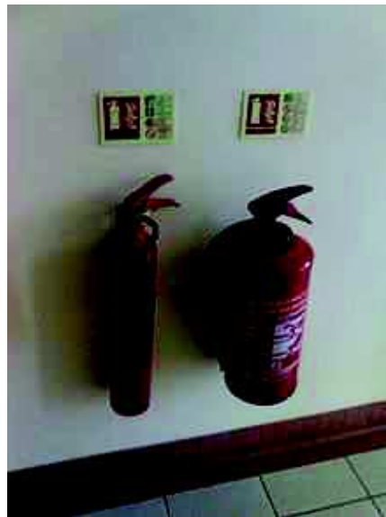
Fig 2.14: Typical United Kingdom CO 2 and water fire extinguishers
