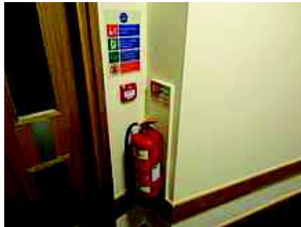
Fig 2.12: A British fire extinguisher with ID sign, call point and fire action sign
