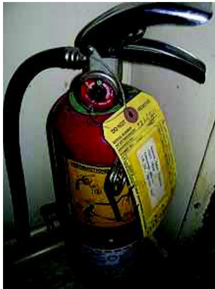
Fig 2.24: An empty fire extinguisher which was not replaced for years.
