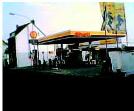
Fig 2.06: A gasoline station.
