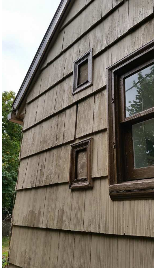
Fig 4.13 Cold pantry exterior vents
