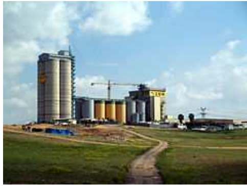
Fig 4.06 Silos connected to a grain elevator on a farm in Israel.
